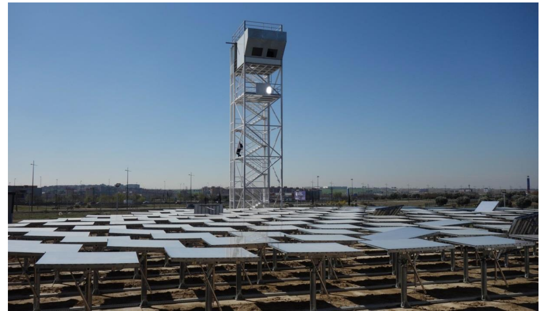
Sun to Liquid Field Demonstrator (Successor of Solar Jet), IMDEA Energía at Móstoles Technology Park, Madrid, Source: Bauhaus Luftfahrt
